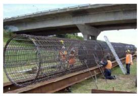
Welding O-cell Assembly to Reinforcing Cage
